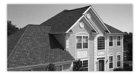
Asphalt shingles are the most commonly used type of shingle across North America. Today's asphalt shingles are reinforced with a fiberglass mat or an organic material such as paper or wood fiber, and can typically range in life expectancy from 10 to 20 years.
