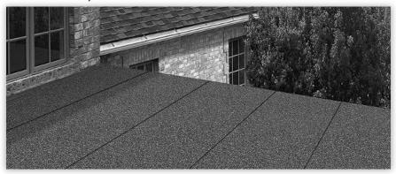
A steep-slope roof (typically a shingle roof) depends upon gravity to cause water to flow in one general direction so it can "shed" the water over the breaks and fasteners in the shingles until it flows to the edge. A low-sloped or flat roof can't depend upon the water to flow in any particular direction so it must form a watertight, monolithic membrane that stays watertight all the way to the drains or edge.
