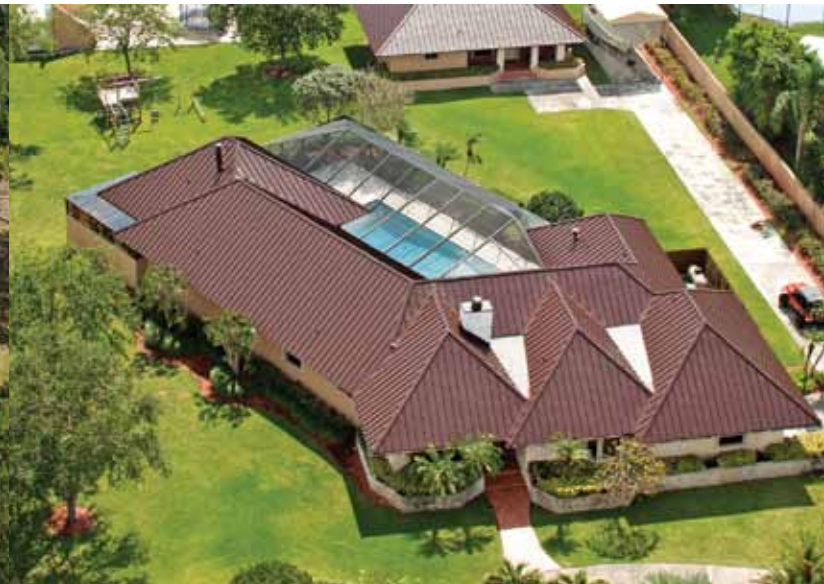
Featuring a contemporary Mansard Brown 1.5 standing seam metal roof, this home's roof was designed and installed with Smart Target details to ensure premium quality and maximum security.
