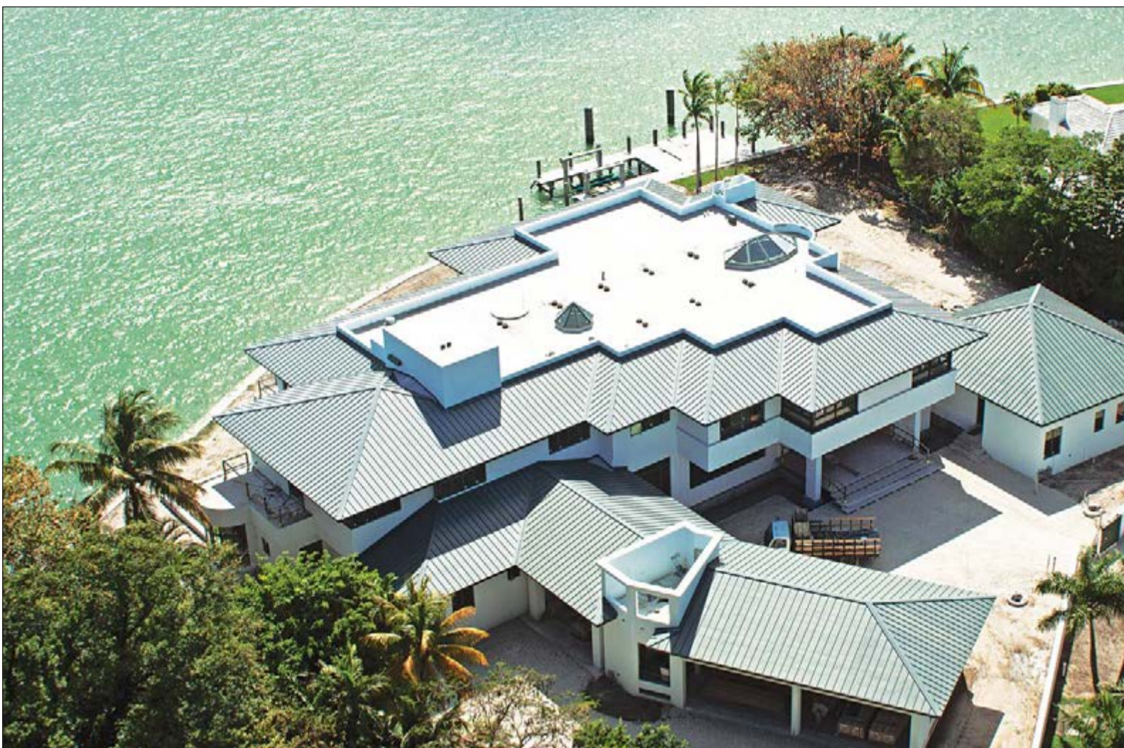
A metal roof is generally considered to be more wind-resistant than shingles or tiles. (Photo courtesy of Istueta Roofing)
