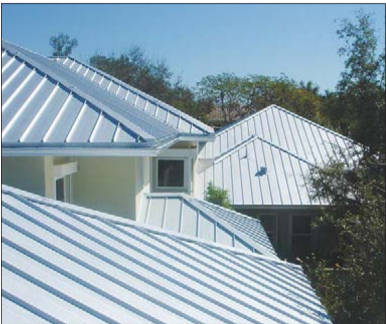
Most residential metal roofs in South Florida are made from either Galvalume or aluminum. (Photo courtesy of Istueta Roofing)
